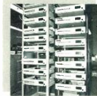
Each Ward-Beck unit seen here will connect an ABC studio with the computer-controlled intercom.
